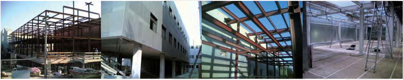
Construction works for the IMB new offices and laboratories building (2005-2006).
